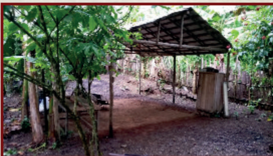
The present carpentry shop, that will be upgraded with a concrete floor and up to date tools.
